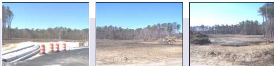
Recently cleared site on Nesbit Road
